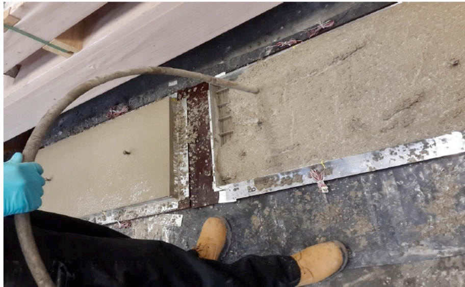
a) Using a manual vibrator to compact the fresh concrete
